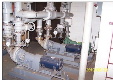
Photo 6 - Existing Heating Hot Water Circulating Pumps
