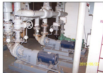
Photo 6 - Existing Heating Hot Water Circulating Pumps
